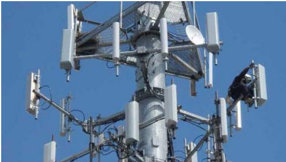
Huawei LTE Base station with several antennas
